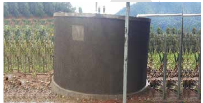
One of the newly constructed rain water harvesting tanks. Photo Credit: Wellard Makambo|IGCP
